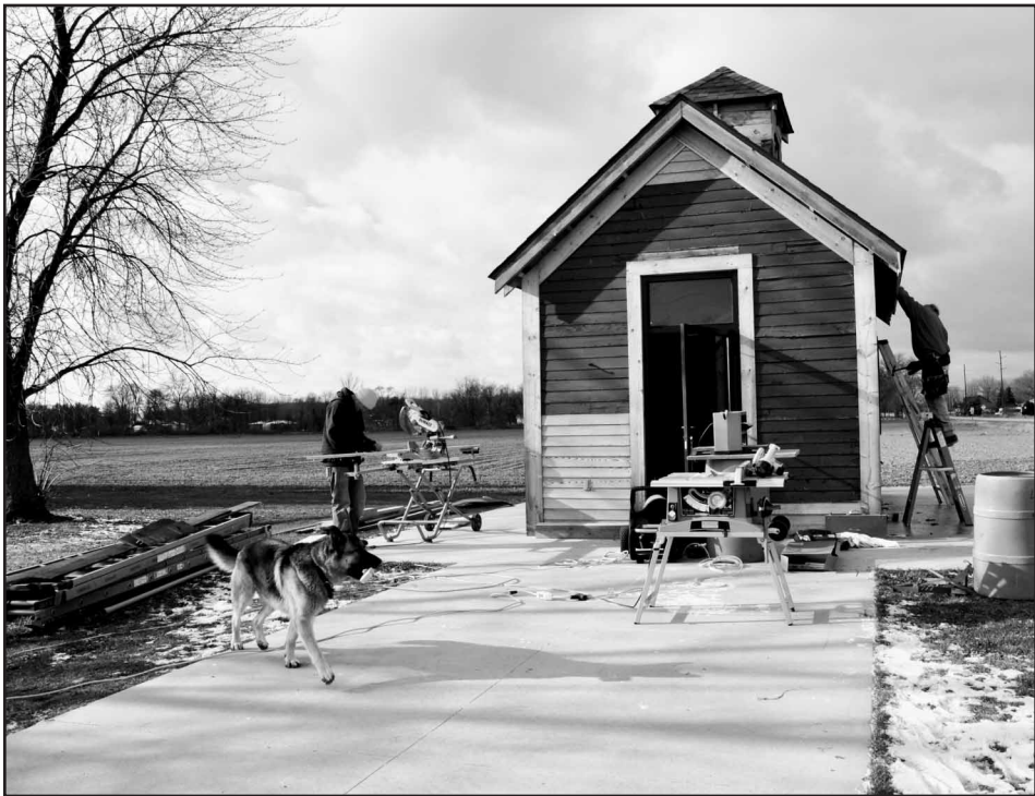
SCOTT CHAMBERS Construction foreman Dave Vigue and employee Nate Hillabrand, shown above, start the finishing touches on the exterior of the Linwood Icehouse Museum last week. Donations of wood, electrical components and money have made the different projects possible. In the foreground is Dave's dog, Ranger, who seems to be earning his keep by carrying one of the smaller pieces of wood.
