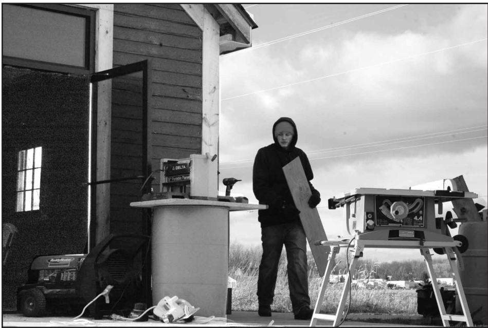
SCOTT CHAMBERS Construction foreman Dave Vigue and employee Nate Hillabrand, replace some of the soffit boards on the Linwood Icehouse Museum, in Linwood, last week. Most of the work on the icehouse has been made possible through generous donations and fundraisers.
